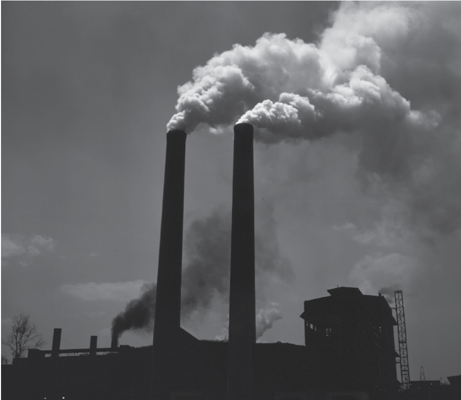
Figure 1. Stacks billowing white ‘smoke’ are often emitting only steam and not polluting the atmosphere with CO 2 or particulate.
